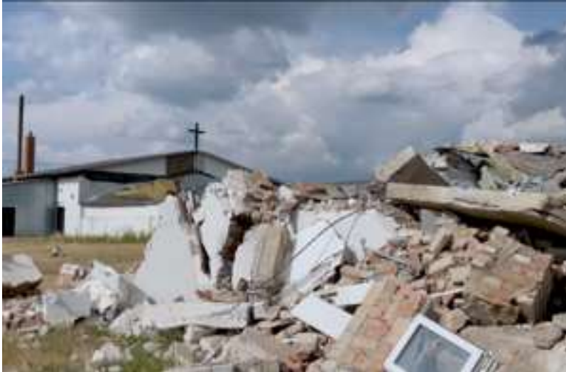
Bulldozed New Life Church, Minsk, 20 June 2023 New Life Church [CC BY-NC-ND 4.0]
