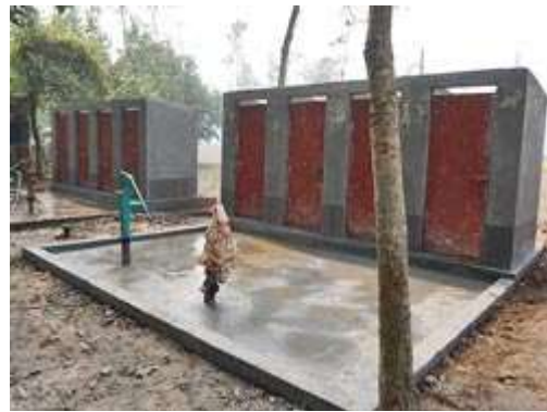
Tubewells with handpumps, and toilets stand ready for the Santal Christians when they move into their new homes
