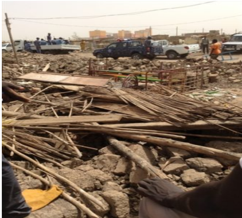
This Sudanese Church of Christ building in Bahri, North Khartoum, was demolished by order of the government on 1 July 2014. (Photo: Open Doors International)
